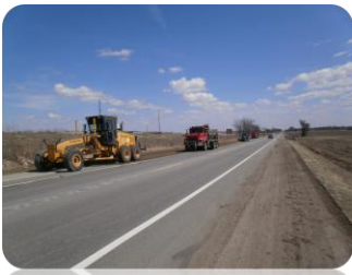
The above photo shows a Road Commission crew from the Grand Haven garage grading shoulders along M-45 with a motor grader.
