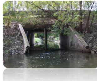
Shown above is the existing timber box culvert at the Brower Drain crossing on Riley Street just east of 104<sup>th</sup> Avenue. The culvert will be replaced with a 15' x 9'
