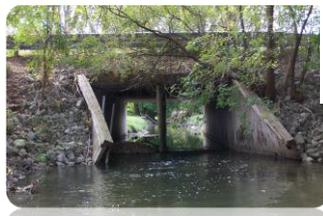
The previous photo shows the condition of the timber box culvert prior to the improvements. The next photo shows the completed Brower Drain concrete box culvert.
