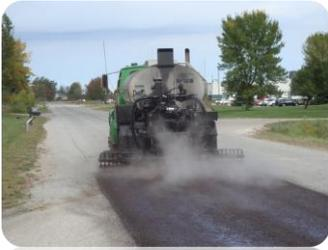
Shown above is a photo of Kent, Montcalm, and Ottawa road crews placing a fog seal over a recently seal coated road.
