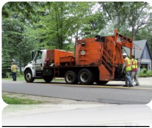
Shown above is crack sealing work performed in 2013 by Scodeller Construction.
