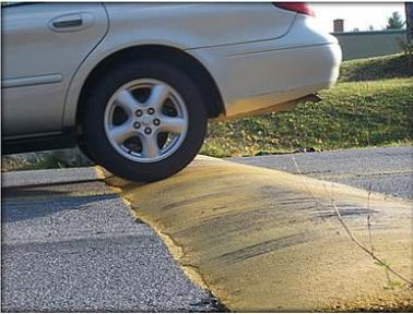
The purpose of a speed bump is to make the ride over it uncomfortable for the driver, encouraging him/her to reduce their speed. With the various vehicle suspensions and wheel bases, the speed bump has shown an inability to successfully control speeds.
