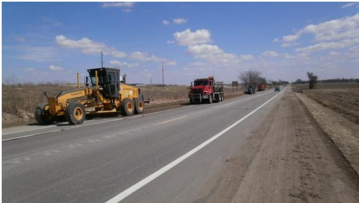
A similar process is done on gravel roads where gravel is displaced onto the shoulder from either rain washing it off the road or from vehicles kicking it up from normal driving. By pulling shoulders on gravel roads and reclaiming it back into the roadway surface, the Road Commission saves thousands of tons of gravel each year.
