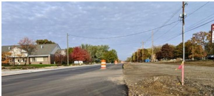
**Reconstruction:** Total removal of the old pavement, aggregate base and sand subbase; utility relocation; then storm drain upgrades, repairs or replacement; then placement of new sand, aggregate and pavement. This is the most aggressive and costly solution to road damage.
