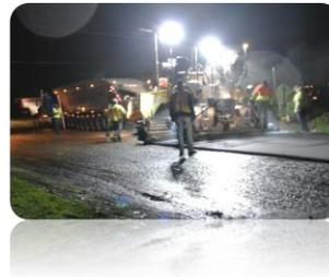
The placement of the asphalt was in accordance with 2012 MDOT Standard Specifications for Construction. During paving, inspectors verified that the surface was prepared properly, the surface temperature was at or above the minimum allowed, and the as-placed asphalt exceeded minimum temperature requirements.
