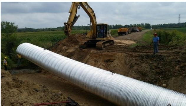
The Stegeman Drain project was located on Van Buren Street between 56<sup>th</sup> and 48<sup>th</sup> Avenues in Blendon Township. The photo to the left shows Hudsonville garage crews installing an Aluminized 87"x63"x60' Corrugated Metal Pipe for the road crossing. The total cost was \$18,700 for the replacement project.
