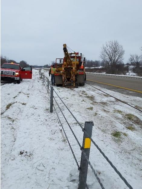
Median cable guardrail consists of steel wire cable mounted on posts. It is designed to prevent a vehicle from leaving the roadway and striking an object which would create a potentially more severe situation. It functions by capturing or redirecting vehicles while absorbing impact energy. With use of this system, MDOT is estimating a reduction in cross-median crashes by 90 percent.
