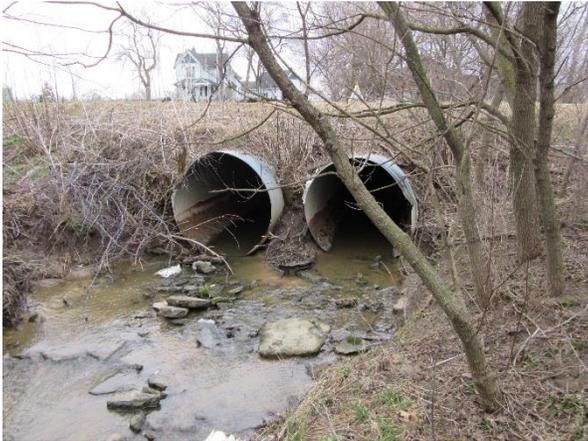
The photo is from 64<sup>th</sup> Ave at Drenthe Creek in Zeeland Township, which flows to Black Creek in the Macatawa Watershed. The outfall has bank erosion on the left side, and the culvert is slightly perched and heavily rusted. With the dual culverts reaching their life expectancy, they will be replaced this year with a single pipe arch recessed below stream bottom which will improve stream flow and function.
