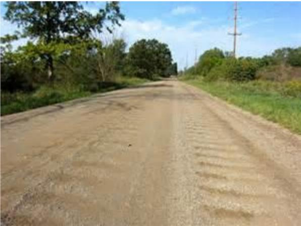
**Lack of moisture.** Prolonged dry weather like we have experienced this summer can cause wash-boarding of the gravel road surface, even with relatively low traffic.
