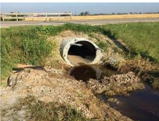
Road Commission crews installed a culvert liner system to rehabilitate a culvert along 96<sup>th</sup> Avenue between Quincy Street and Riley Street as a pilot project. The final results are shown on the photo to the left. Most of the work was done off the shoulder of 96<sup>th</sup> Avenue, which provided a safer environment for the work crews and motoring public. The cost for the work was approximately \$27,000 which was determined to be comparable to a complete culvert replacement cost.
